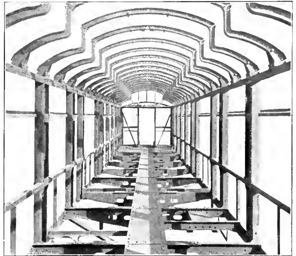
Interior View Showing the Details of the Body and Underframe Construction
